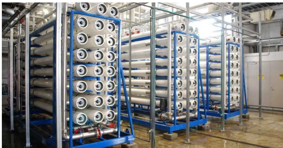
A WesTech Reverse Osmosis System rated for 2,000 gpm capacity.
